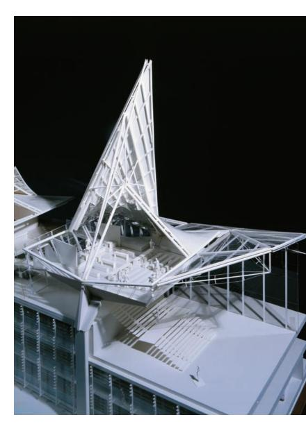
grid. This grid of beams in turn was covered with LVL kerto plywood to form the outer structural skin of the roof.
