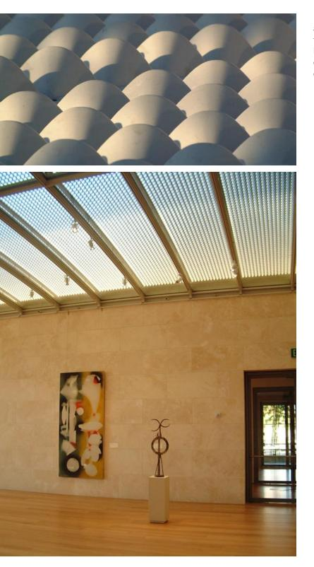
The innovative use of 3-D computer modelling and rapid prototyping enabled the development of this unique shading product optimised for the site. It enabled good communication with the client and design team and dramatically reduced the time from concept to manufacture.
